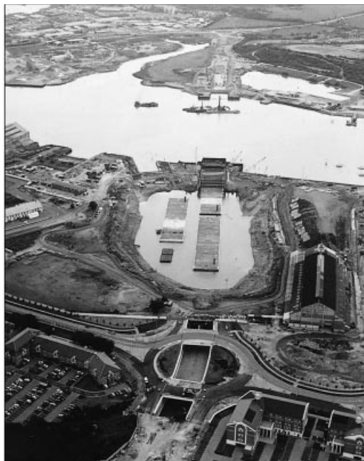
Fig. 8. Immersed tunnel elements in partially flooded casting basin
