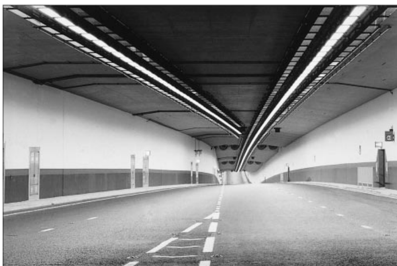
Fig. 17. View of mechanical and electrical installations, including jet fans in ceiling niches and enhanced lighting at tunnel portal
