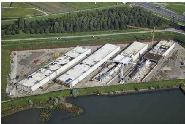
Figure 1. Tunnel elements in the Barendrecht casting yard.
